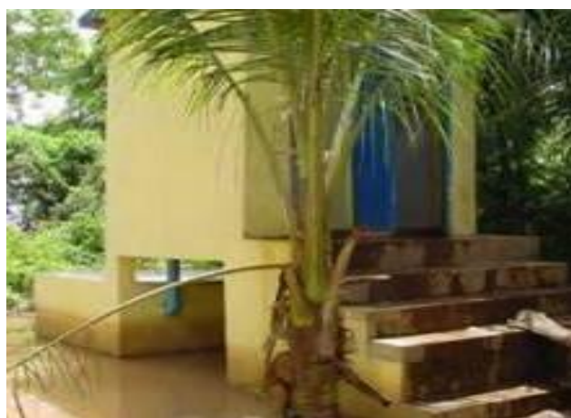
Examples of raised off-set communal latrines, with single or double pits
