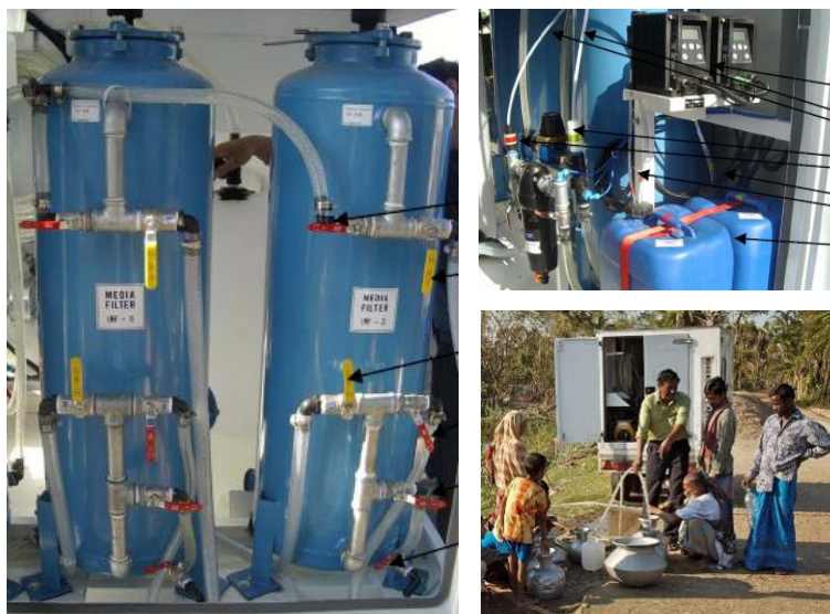
An example of UNICEF-DPHE mobile treatment plant, installed in a vehicle for easy transport and installation.
